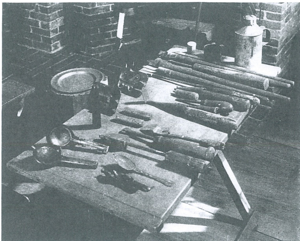
Tools of the pewterer Samuel Pierce, 1767-1840, of Greenfield, with spoon molds and spoons. A pewter plate rests on a wooden chuck used to shape the piece in spinning. Note the insulating corncob handle on one of the soldering irons. The face of Pierce's iron die, which stands upright in foreground, is shown in detail at the right. Hall Tavern
