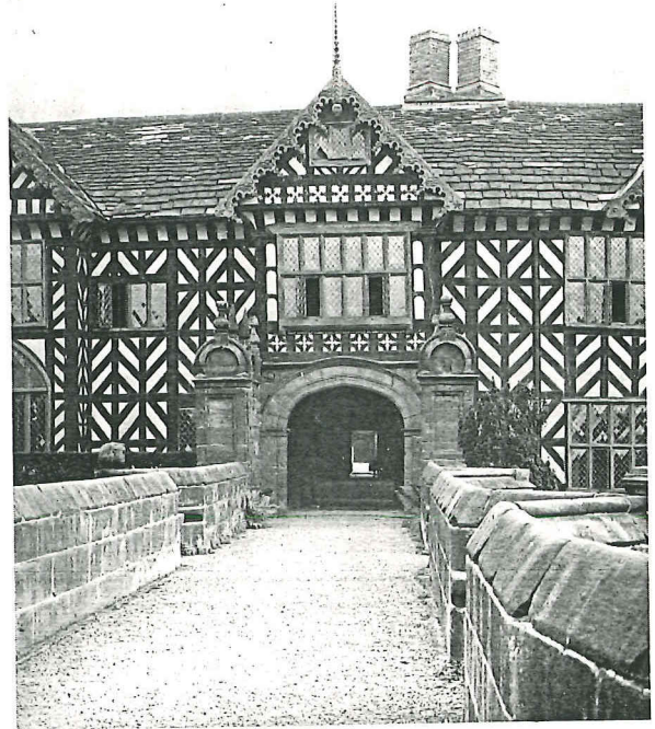
SPEKE HALL. North Porch and Bridge
