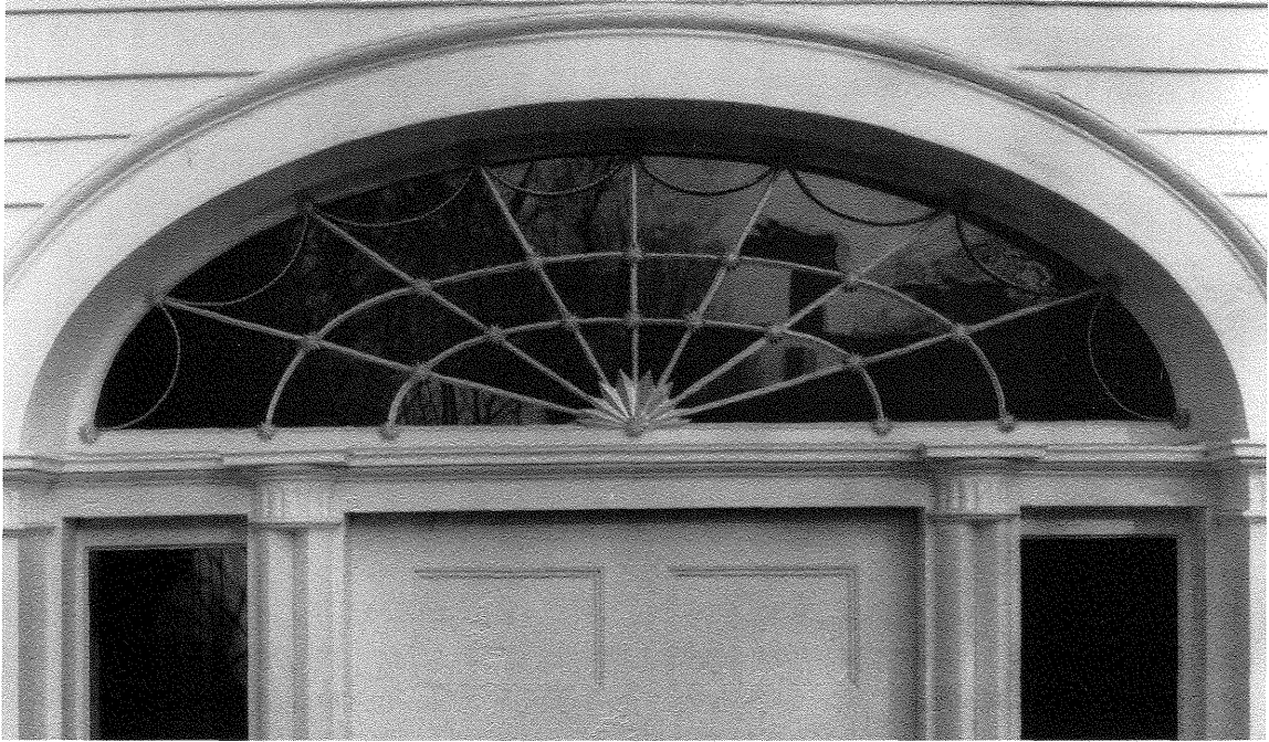
Fig. 9. Fanlight, Hinsdale and Anna Williams House, Deerfield, MA., about 1816. Glass, white pine, and lead. H: 22 1/2". Photography by Amanda Merullo. Although written documentation has not survived, the beaded, lead swags and gilded rosettes that ornament the neoclassical doorway of the Williams House match the wooden molds found among Pierce's tools. Pierce and the Williams family lived three miles apart.
