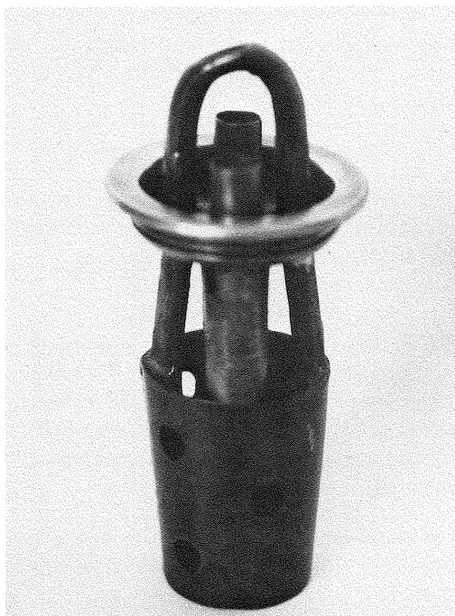
Fig. 2 Heating element found in a Sellew type whale oil lamp.
